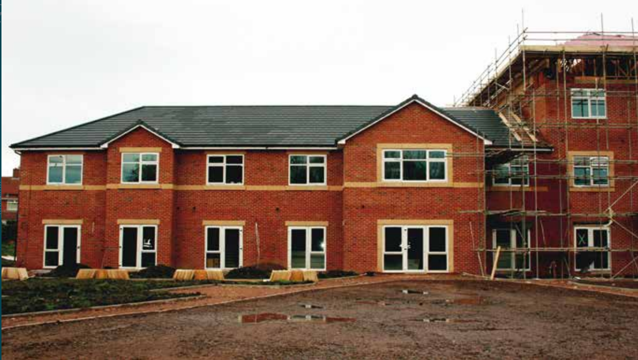
Construction well advanced on Wallsend site
